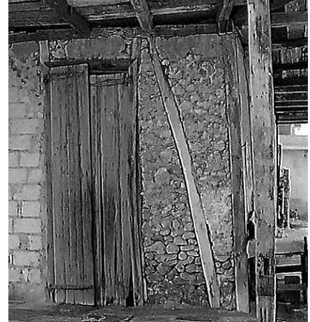
Right: detail of a traditional braced wood frame with infill
