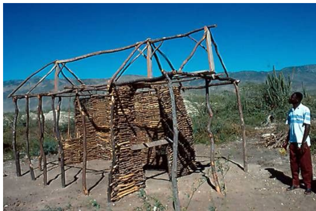
Left: traditional woven panel construction
